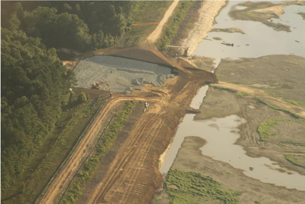
Aerial view of the Woodlake dam being demolished earlier this year
